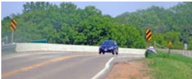
The I-94 overpass along 141st Ave. N. provides a critical east/west connection over a major physical road barrier.
