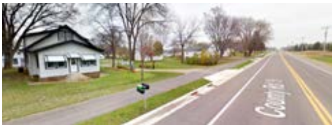
Constructed adjacent to CR19, the new CRRT portions connect downtown Hanover to Crow-Hassan Park Reserve's southern end and Lake Independence RT.
