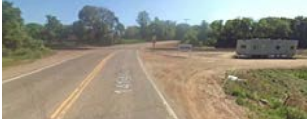
An at-grade railroad crossing poses a CRRT challenge due to the horizontal curve along 141st Ave. N.
