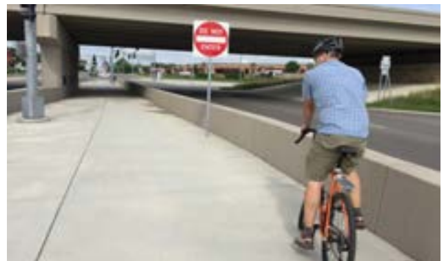
Bicyclist correctly utilizing the center refuge island of the 141st Ave N. diverging diamond interchange.
