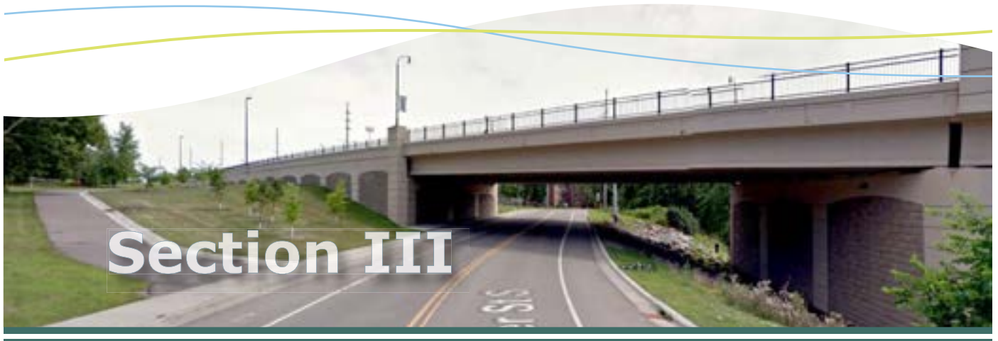
CRRT Character CRRT's connection to Highway 12/Babcock Blvd. and River St., Delano, MN Image Credit: Google Streetview
